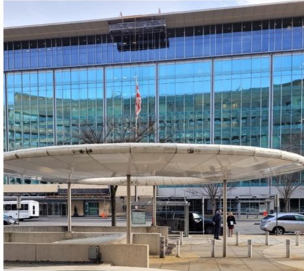
Air handler units are 29 years beyond useful life. Replacement needed for reliability, indoor air quality, and streamlining of repair costs.
